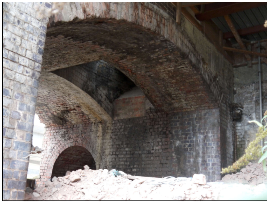
EXISTING PARTIALLY COLLAPSED VAULTS CONNECTED TO LISTED VIADUCT ON BRAITHWAITE ST TO BE REMOVED.
